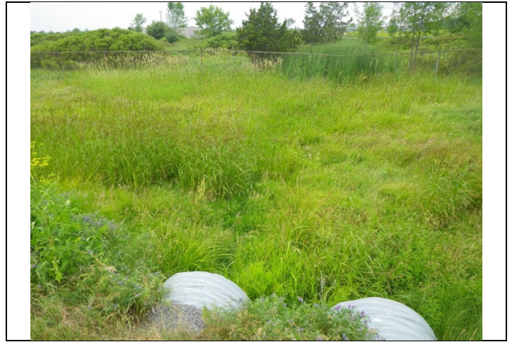
Photo 14 M5 – Facing upstream from Taylor Kidd Boulevard showing channel overview.
