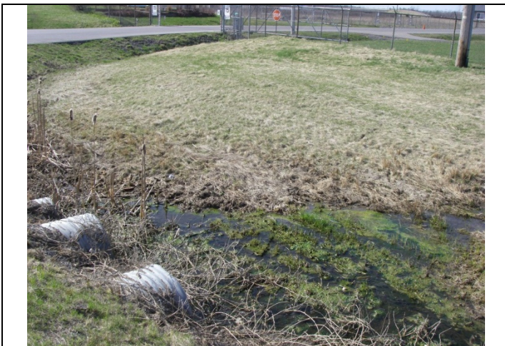
Photo 9 M4 – Facing upstream from Taylor Kidd Boulevard showing lack of channel.
