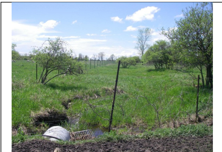
Photo 5 Station 29 – upstream view from farm crossing of surficial drainage. Some erosion was noted and is a result of an under-sized culvert at the access road
